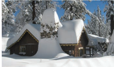
Heavy snow and ice damming can weigh down your roof potentially causing water leaks or worse.
