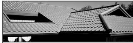
New metal roofing products engineered to resemble other types of roofing have broadened the popularity of metal as a roofing material.
